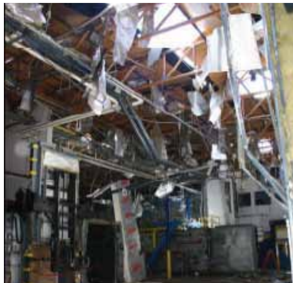
Figure 5.26 Sterilization Chamber Damage
