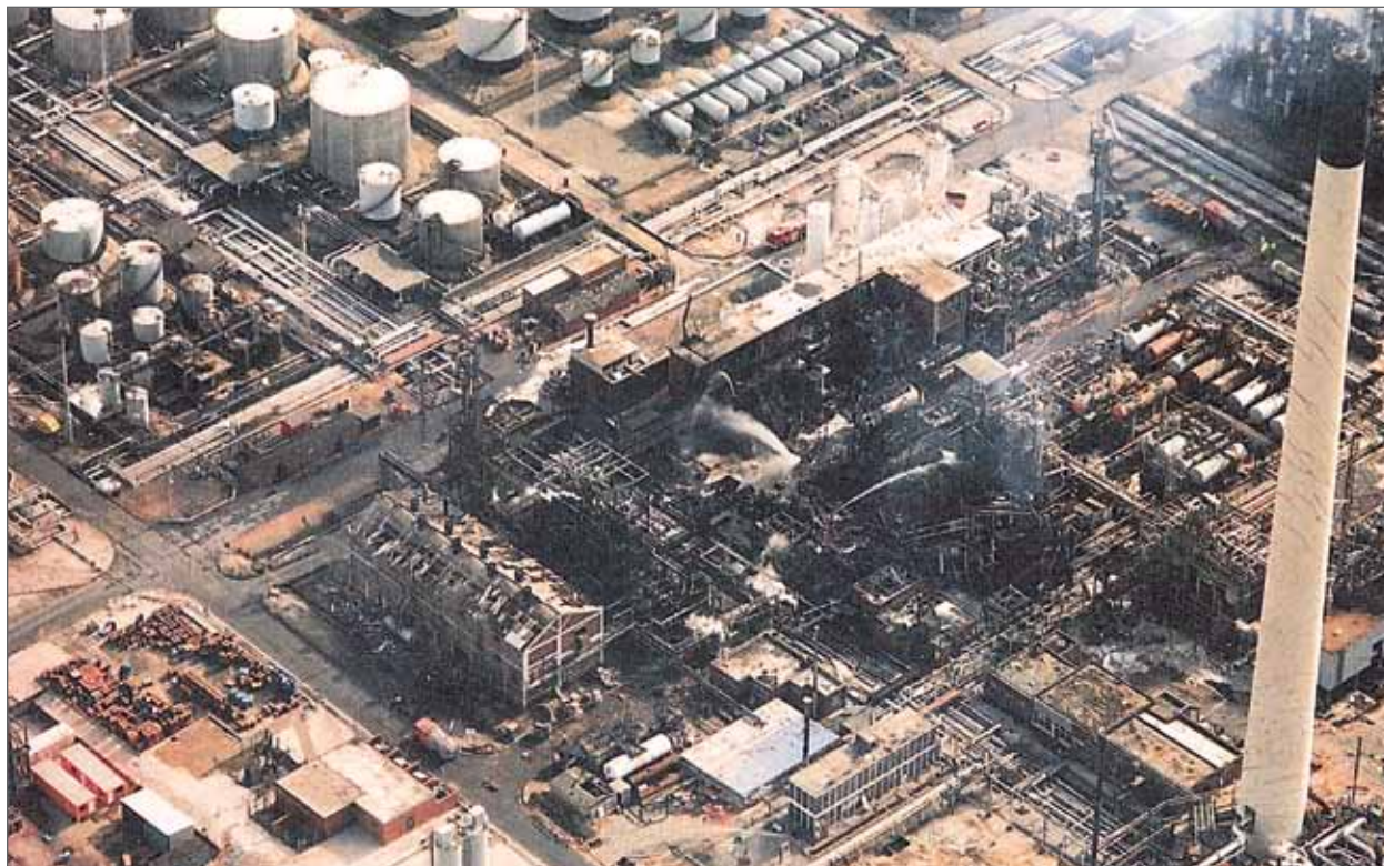
Figure 5.13 Aerial View of Ethylene Oxide Plant after Explosion
