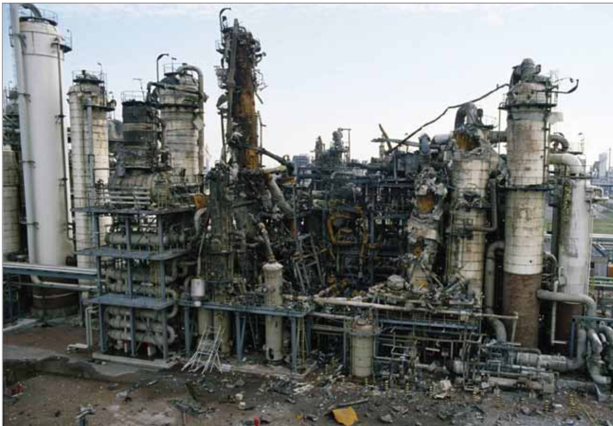
Figure 5.18 EO Purification After Explosion – Two Towers are Missing
