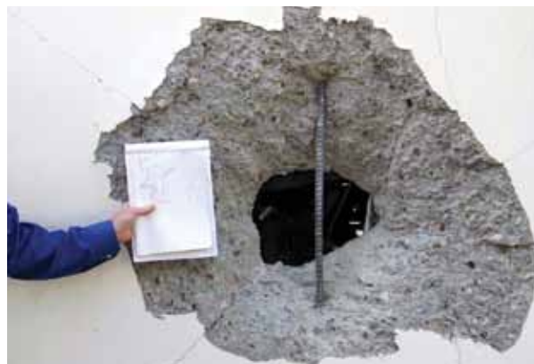
Figure 5.27 Damage to the building wall from impact of sterilizer door
