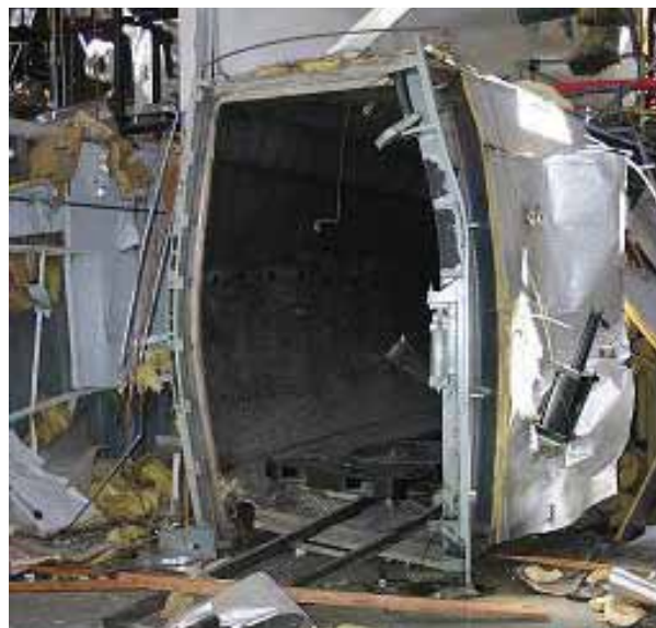
Figure 5.27 Damage to the building wall from impact of sterilizer door
