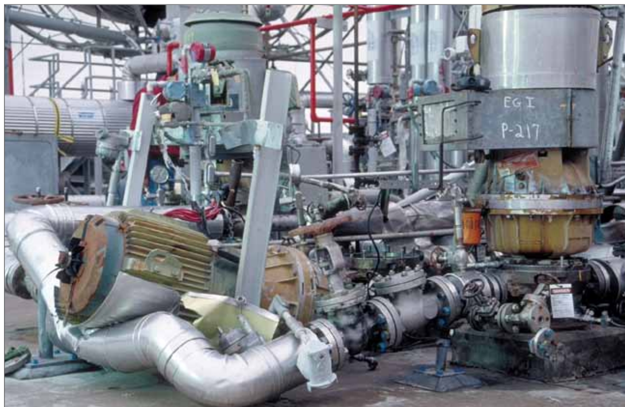
Figure 5.11 Motor Landed on Operating Ethylene Oxide Pump Discharge Line
