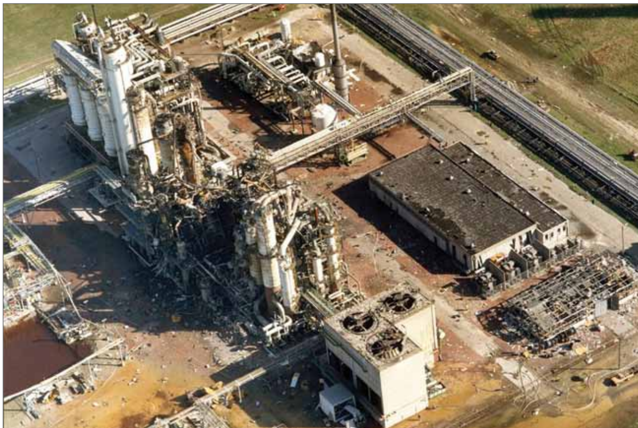
Figure 5.17 EO Plant Burning after Explosion
