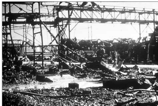
Figure 5.2 Blast Center after Explosion – EO Vessels No Longer Visible
